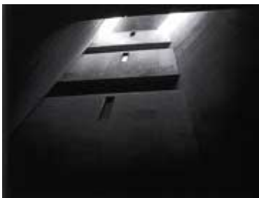
View of one of the voids. Photo: Stephan Freid.
